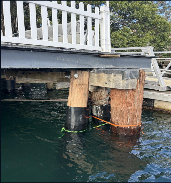
Pile reinforcement
