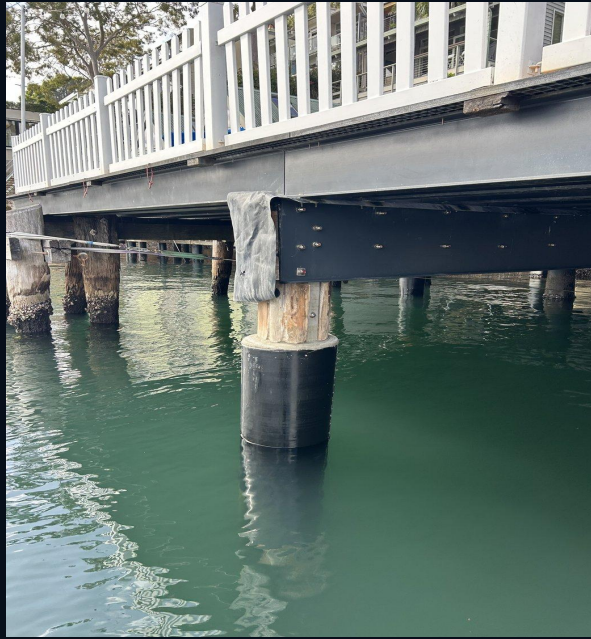
Sleeve installation
